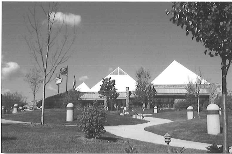
Exterior View Facing Parking Lot
