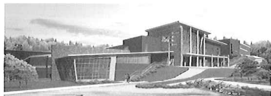
Greenbrier West High School Addition/Renovation
