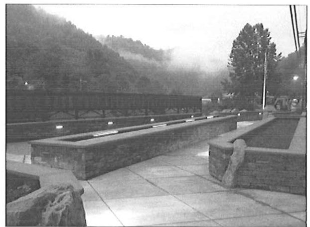
Construction photo prior to installation of granite monument and landscaping.
