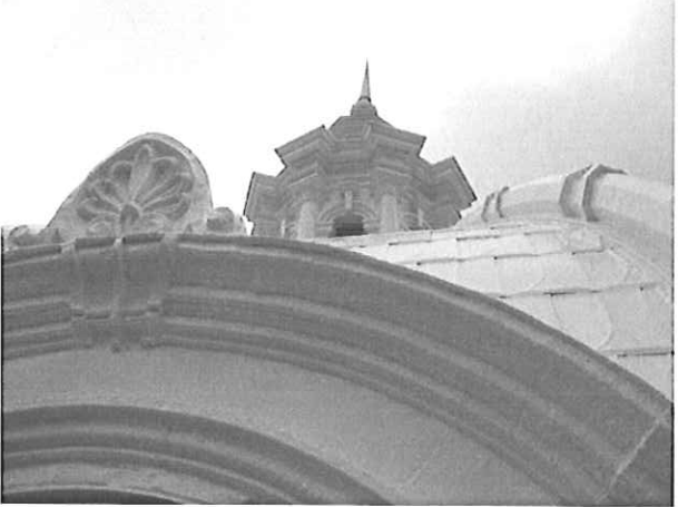
Dome Restoration Detail
