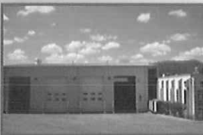
North View Fire Station Clarksburg, WV
