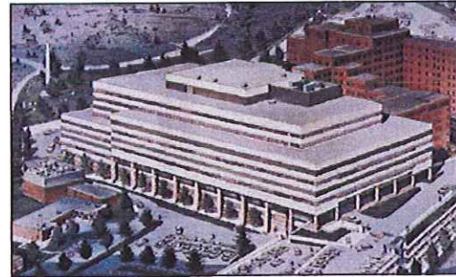
VAMC Philadelphia. Our relationship with VAMC Philadelphia began with a comprehensive master plan and preliminary and final design of a $105 million new construction project.
