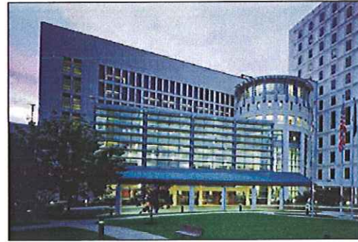
Altoona Hospital. The addition and renovation project received a Vista Award Honorable Mention presented by the American Society for Health Care Engineering.
