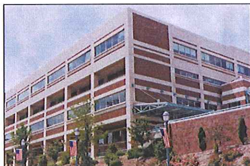
Conemaugh Memorial Medical Center. A new emergency trauma center, pharmacy and maternity ward are part of the five-story, 250,000 sq.ft. addition.
