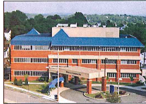
Westmoreland Medical Office Building. H.F. Lenz Company provided the complete base building mechanical/electrical design for this new 40,000 sq.ft., four-story medical office building.
