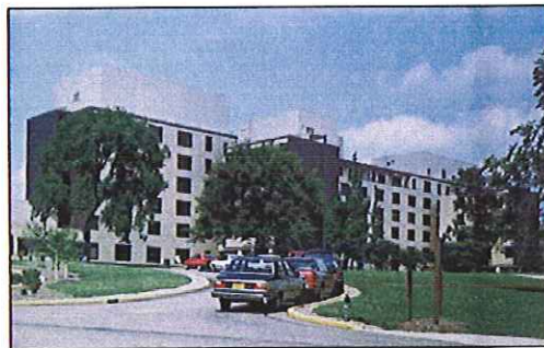
VAMC Highland Drive. The $38 million renovation project was completed under budget and six months ahead of schedule.
