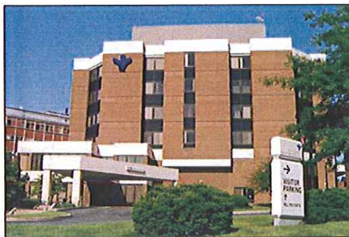
Bon Secours Holy Family Regional Health System. H.F. Lenz Company has completed approximately 80,000 sq.ft. of renovation projects throughout the entire hospital facility
