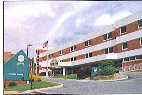
Somerset Hospital. The new addition includes an MRI suite and outpatient surgery facilities.
