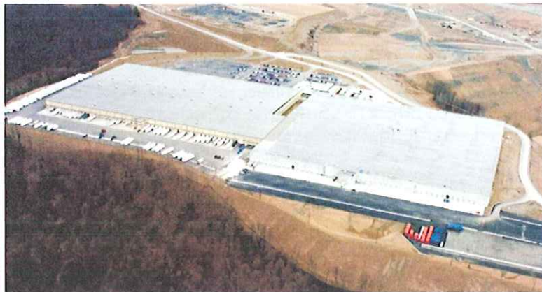
Cabela’s Eastern Distribution Center
