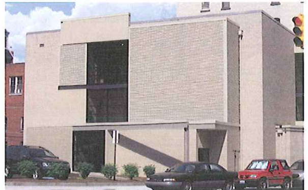
Dr. Ganzer Office Building
