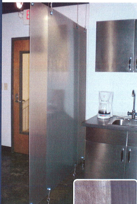
Close-Up of an Airline Cable Anchoring the Kitchenette's Hanging Sheet Metal Wall
