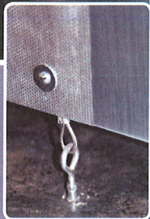
Close-Up of an Airline Cable Anchoring the Kitchenette's Hanging Sheet Metal Wall
