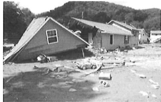
Houses damaged in Clear Creek, West Virginia Flood
