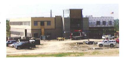
GAI was responsible for site design and permitting, including utility infrastructure design (public water system, storm and sanitary sewers) and access road design. GAI also prepared a traffic study to evaluate the project's impact on the local roadway network. GAI's environmental assessment of the site addressed topography, geology and soils, cultural resources, wetlands and floodplain, and existing utilities.
