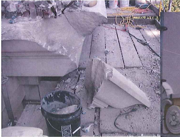
Portions of the limestone cornice were damaged to the point that they fell when work was being conducted and had to be pinned back in place.
