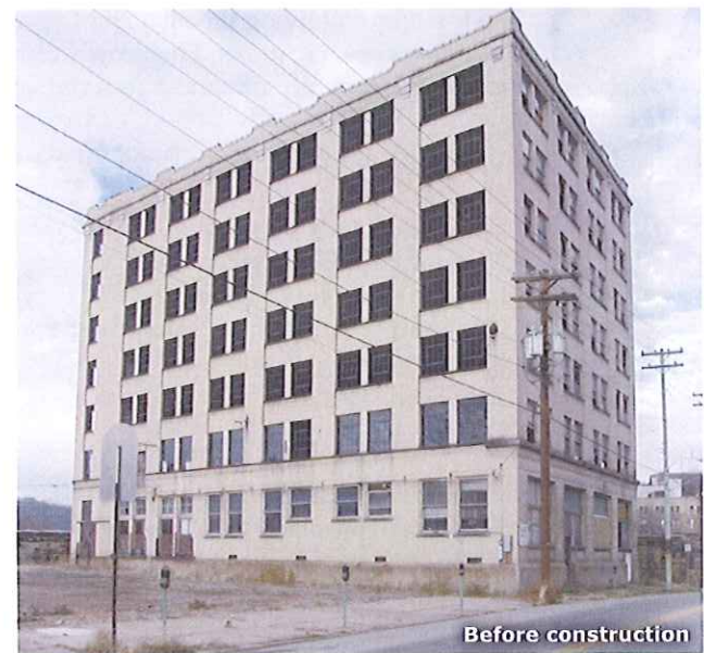
Before demo of adjacent building
