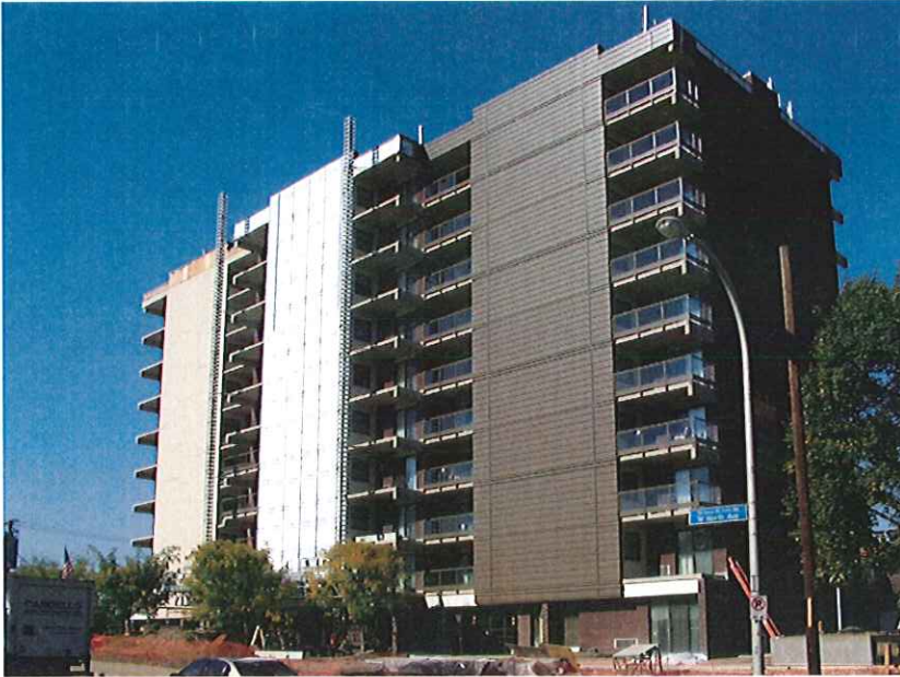
West Park Court during re-skinning of original EIFS exterior (Pittsburgh, PA)
