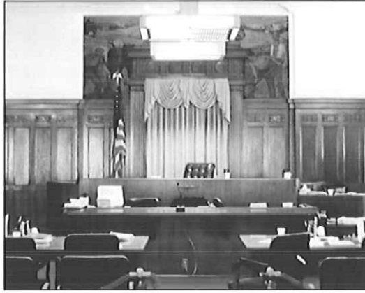
Scranton Courthouse. The project included renovation design for two federal district courts in the existing building.
