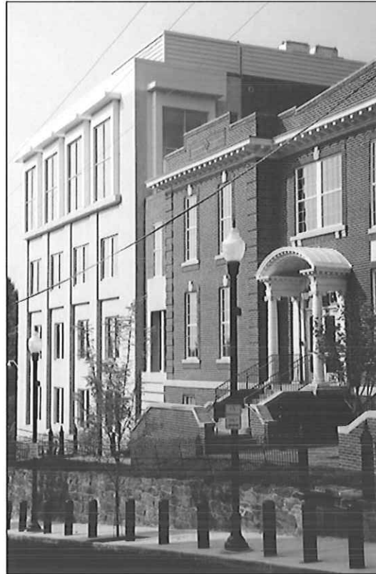
Lynchburg Courthouse. The project was designed to meet the anticipated space requirements of 2010 for the US District Court, US Bankruptcy Court, and several federal agencies, while also providing a new consolidated retail facility for the Postal Service.
