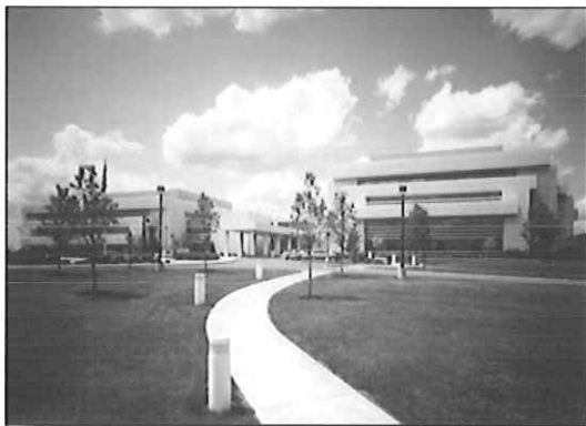
FedEx Ground. The new corporate headquarters contains a raised-floor computer area, an auditorium, a cafeteria, a media production studio, and a fitness center.
