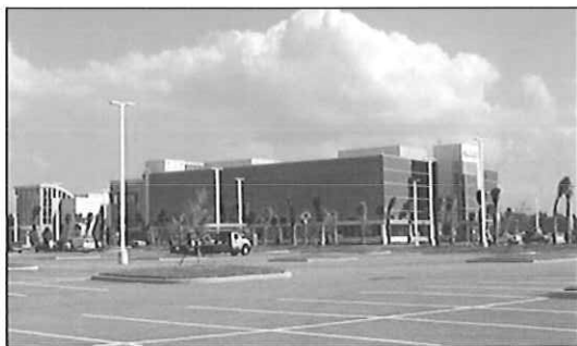
Confidential Insurance Company. The new South-Eastern United States call center building includes employee amenities such as food service, meeting rooms, and training facilities.
