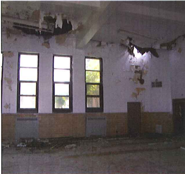
Existing conditions in the Gymnasium/Stage area
