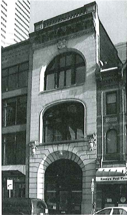
PWWG's office in a former City firehouse in downtown Pittsburgh
