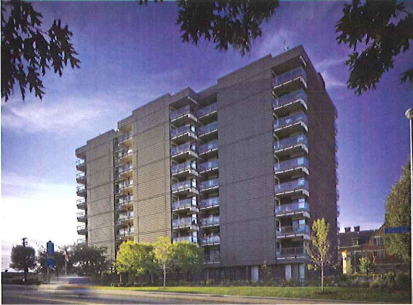
PWWG's re-skinning of a 1970's residential tower at West Park Court
