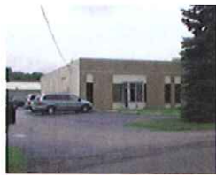
Facility before additions at front, rear, and roof
