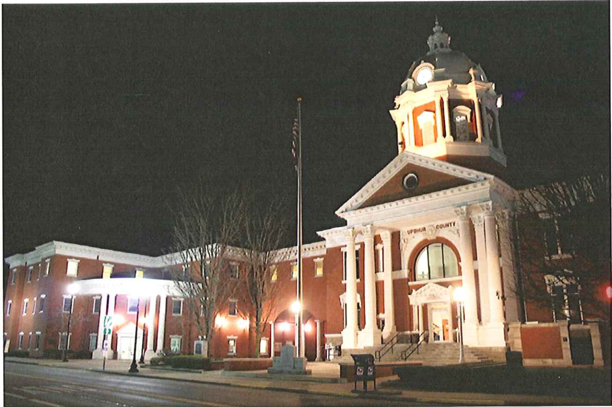
Upshur County Courthouse Complex
