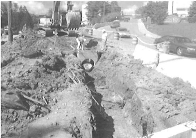
Fairmont State University Storm Water project
