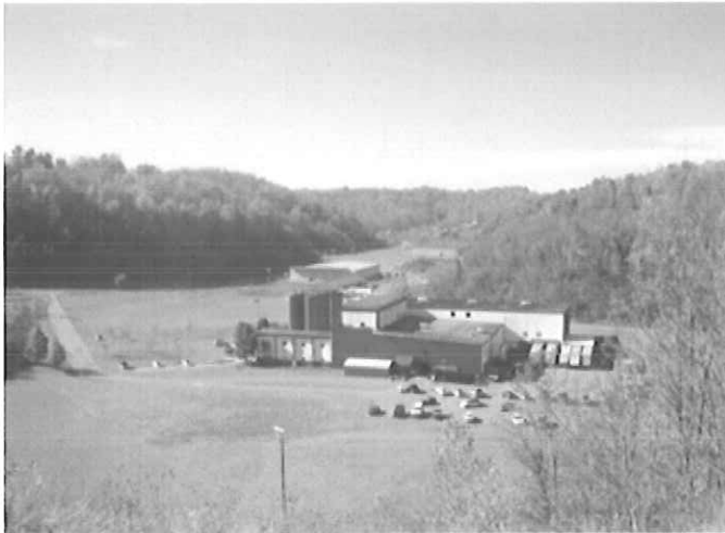
Harrison County Business and Technology Park
