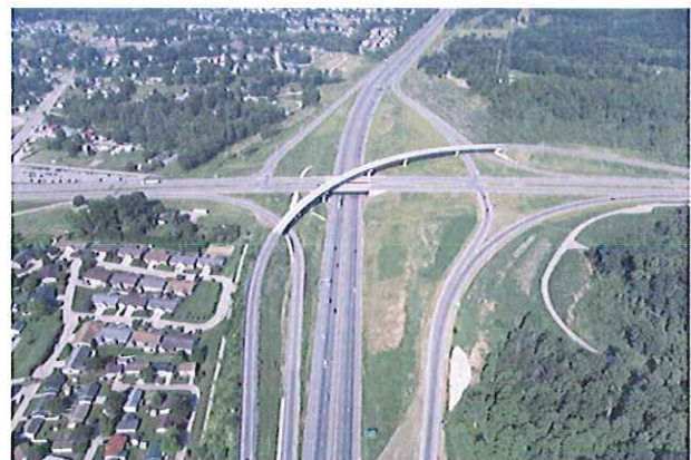
TERRADON provided survey and mapping services on the Route 35/I-64 Interchange as part of a Value Engineering solution through Kanawha Stone Company for the WVDOH. The photo above shows the finished interchange.
