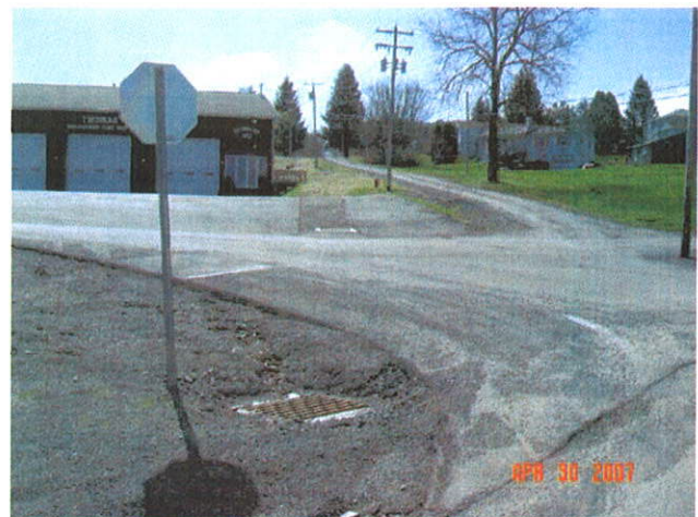
New Storm Drains and Catch Basins
