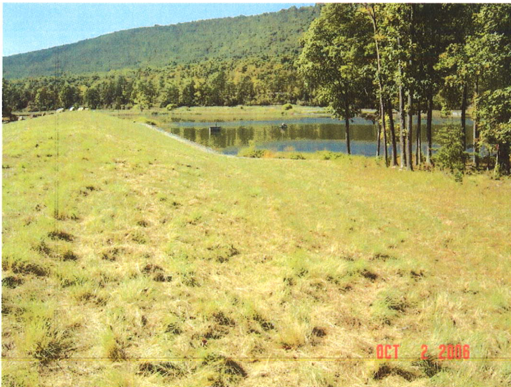
WARDEN LAKE DAM MODIFICATION, HARDY CO., WV
