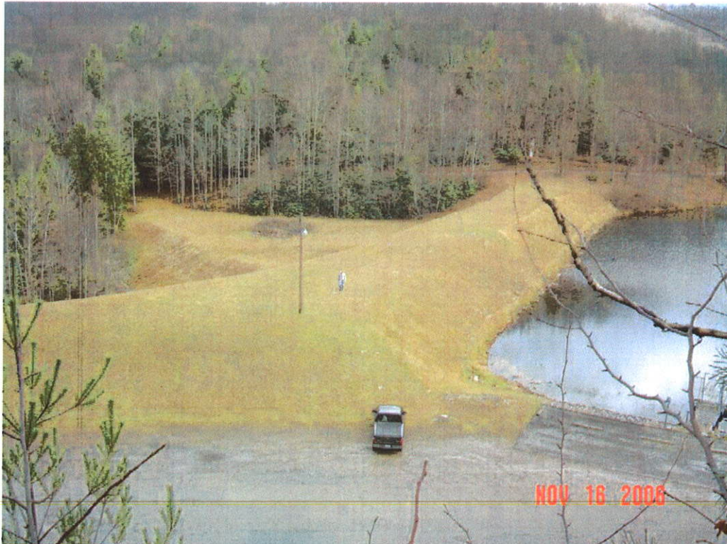
PLUM ORCHARD DAM MODIFICATION, FAYETTE CO., WV
