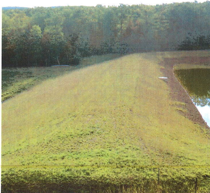
WILSON DAM MODIFICATION, HAMPSHIRE CO., WV
