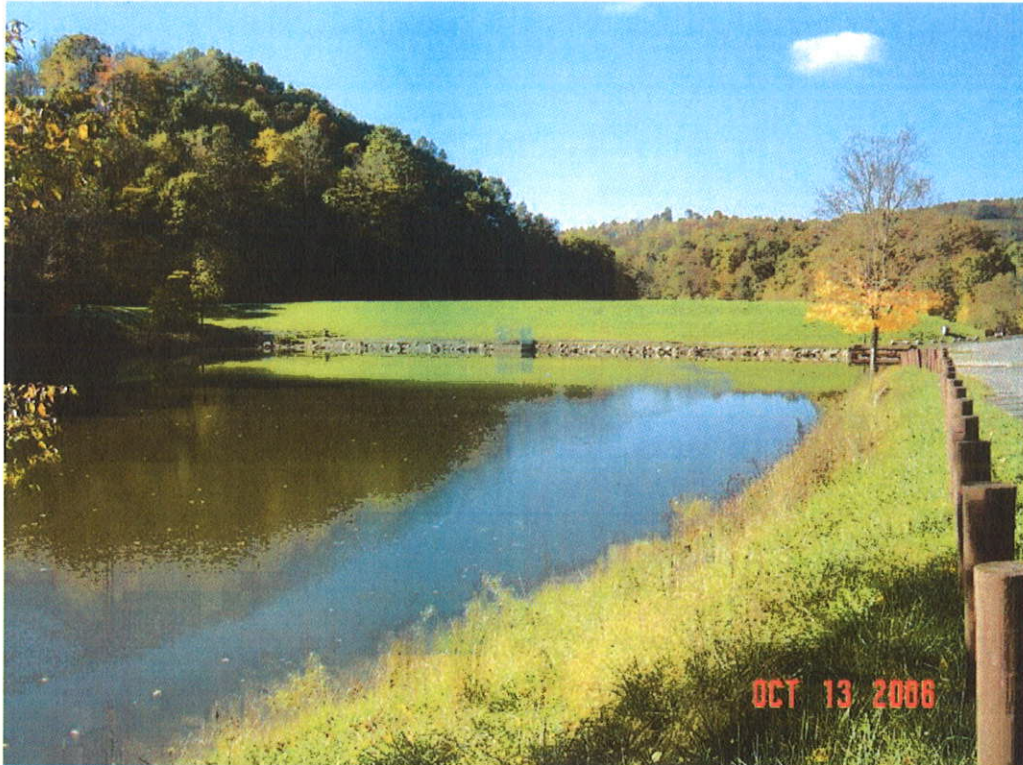
JIMMY LEWIS DAM MODIFICATION, MERCER CO., WV
