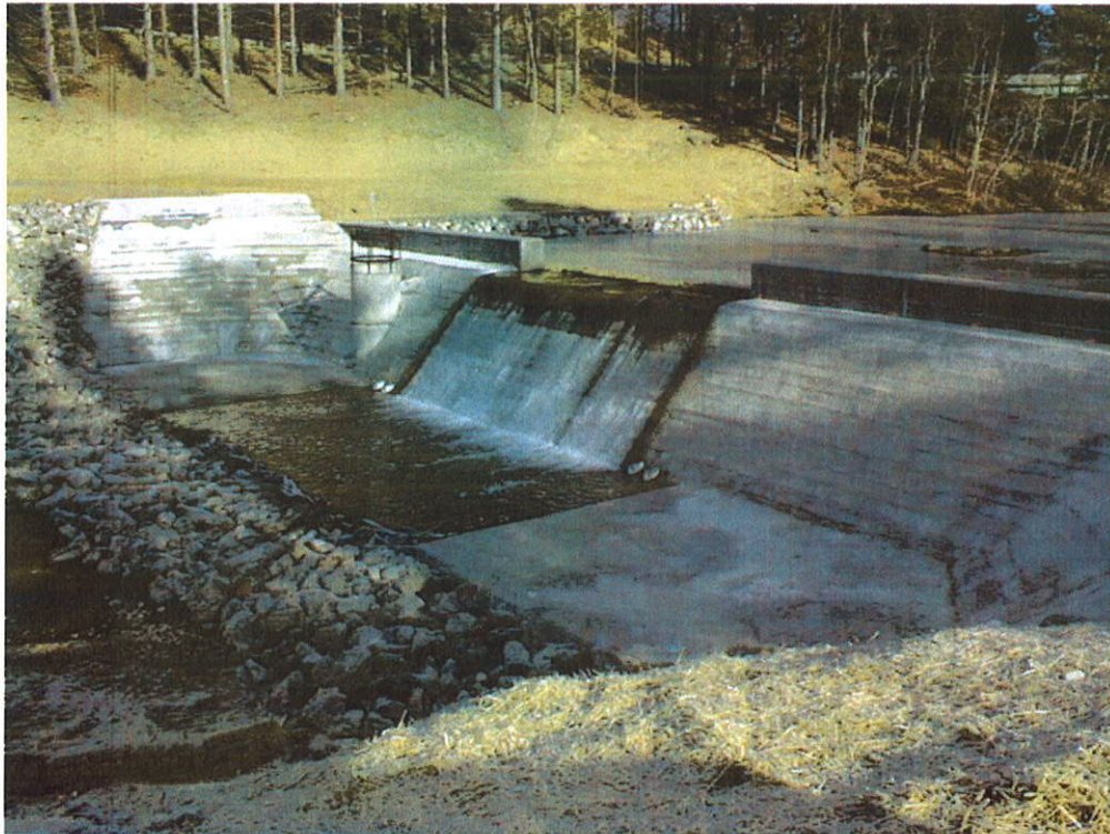
THOMAS DAM MODIFICATION, THOMAS, WV
