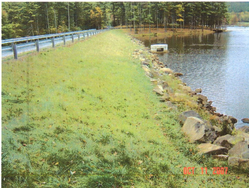
MONCOVE DAM MODIFICATION, MONROE CO., WV
