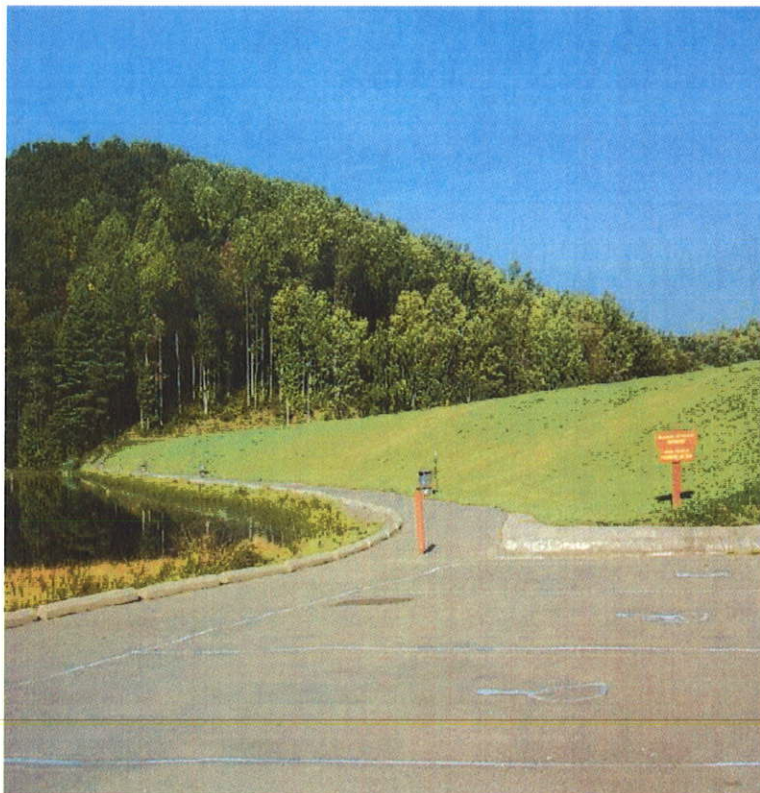
TETER CREEK DAM MODIFICATION, BARBOUR CO., WV
