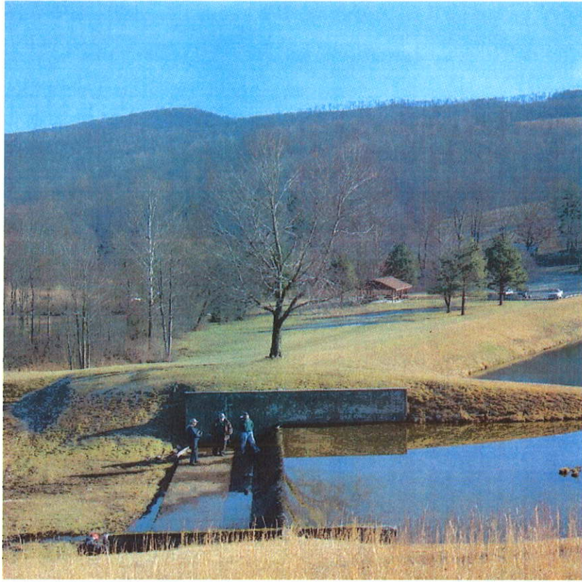
BELINGTON DAM MODIFICATION, BELINGTON, WV
