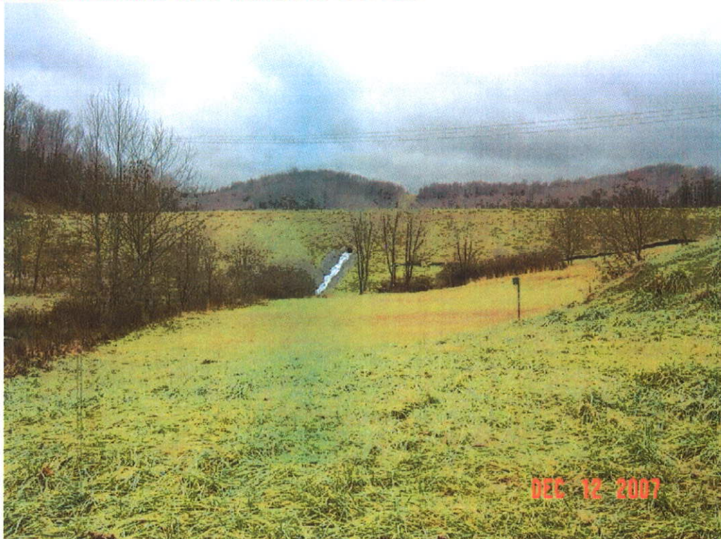
LEMLEY DAM MODIFICATION, MONONGALIA CO., WV
