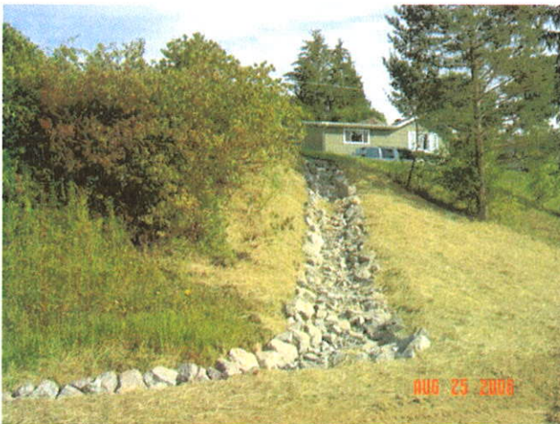
Erosion Repair – Rip Rap Armored Ditch
