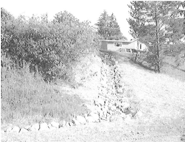
Erosion Repair – Rip Rap Armored Ditch
