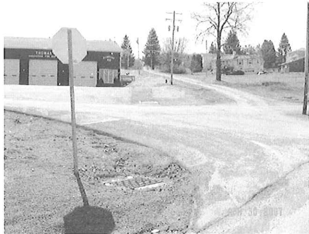
New Storm Drains and Catch Basins
