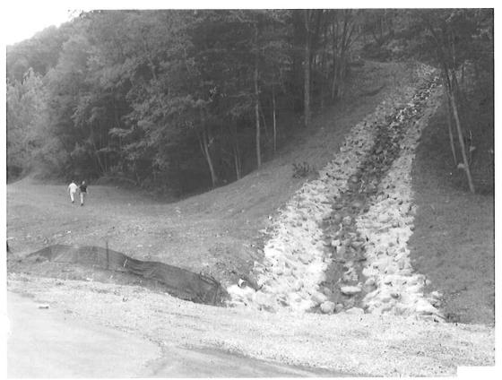
TERRADON has the experience and personnel to handle the wide array of problem areas associated with AML projects. This photo was taken from our Sarah Ann (Vance) project in Logan County, and shows the constructed grouted rip rap channel conveyning drainage from the wet sealed portals located on the bench above.
