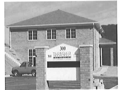
Thrasher Engineering, Inc. Office – Charleston, WV
