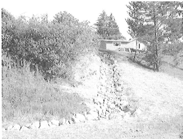
Erosion Repair – Rip Rap Armored Ditch
