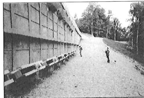
Finished wall with anchors
