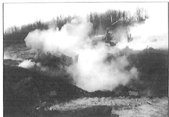
Jamison Burning Refuse Reclamation Project
