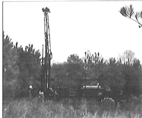
CTL's ATV can drill in rough terrain
