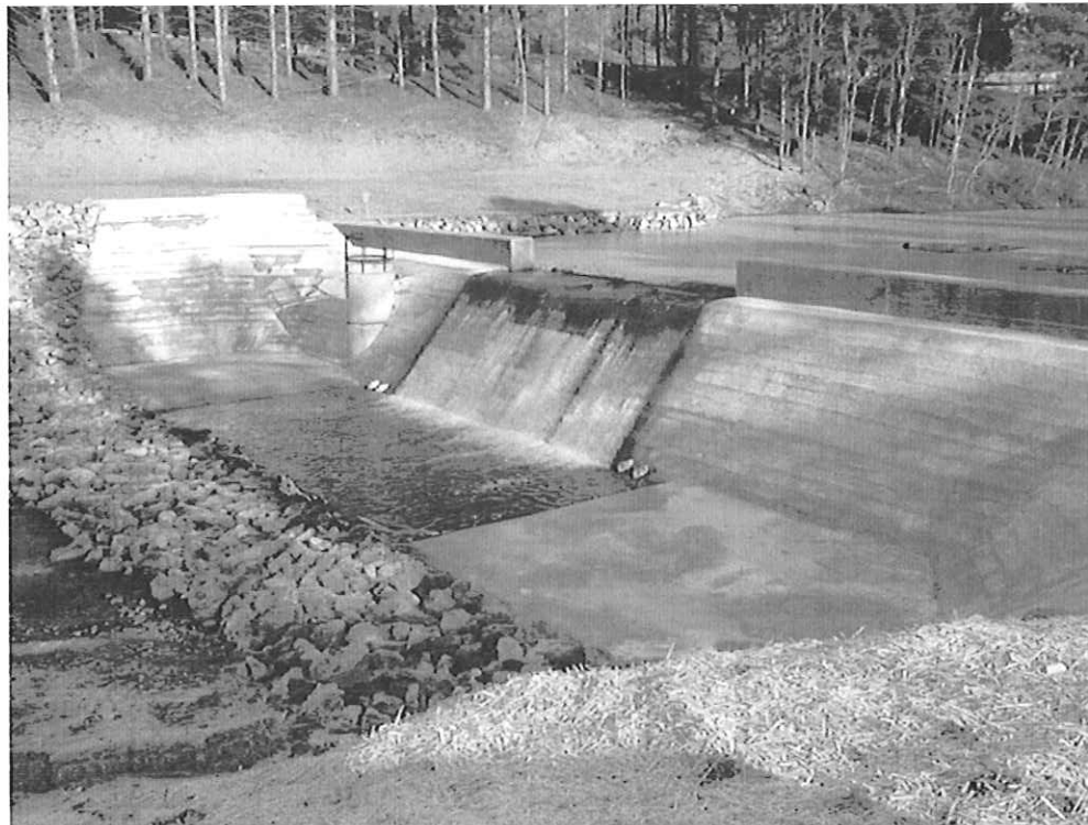
THOMAS DAM MODIFICATION, THOMAS, WV
