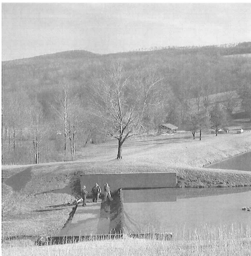
BELINGTON DAM MODIFICATION, BELINGTON, WV
