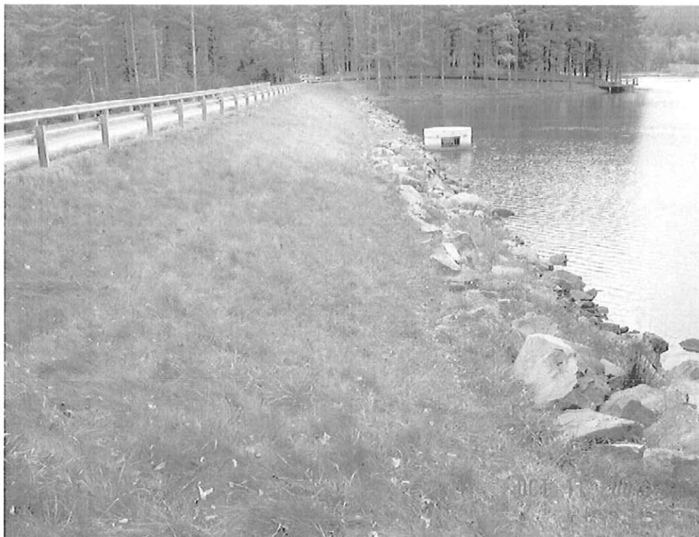
MONCOVE DAM MODIFICATION, MONROE CO., WV
