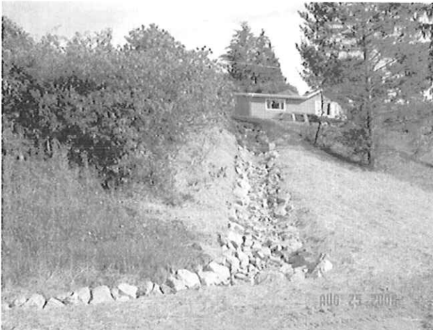
Erosion Repair – Rip Rap Armored Ditch
