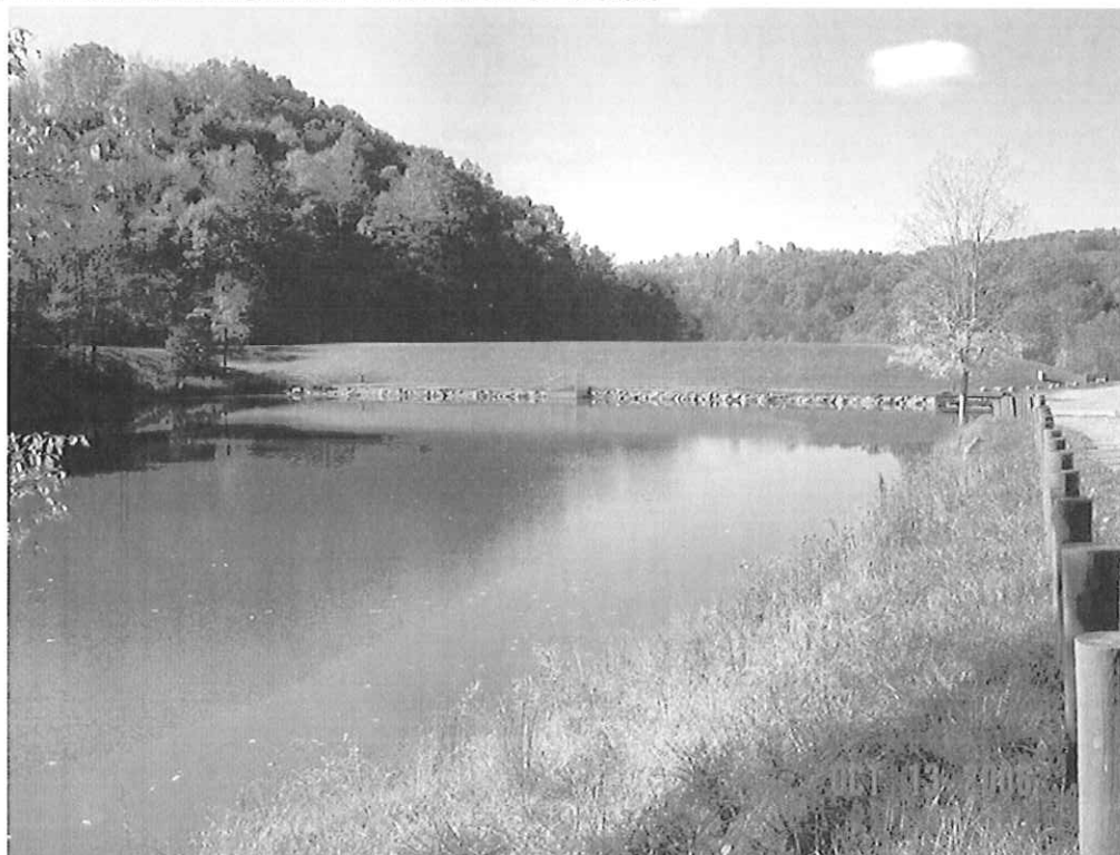
JIMMY LEWIS DAM MODIFICATION, MERCER CO., WV
