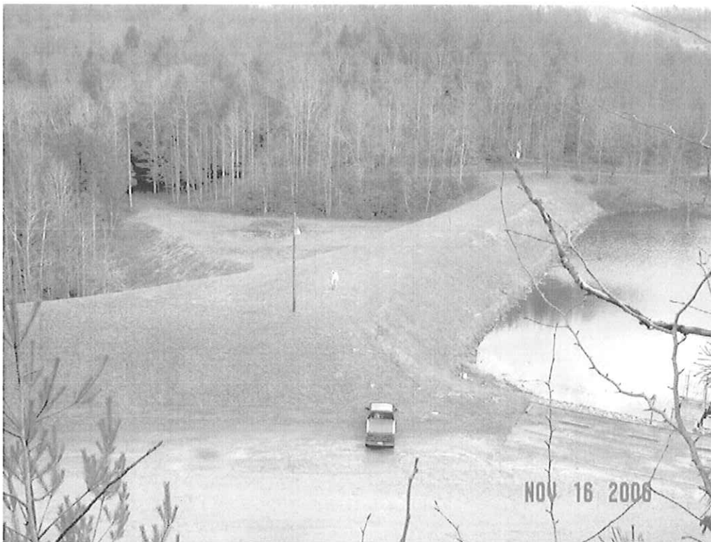
PLUM ORCHARD DAM MODIFICATION, FAYETTE CO., WV
