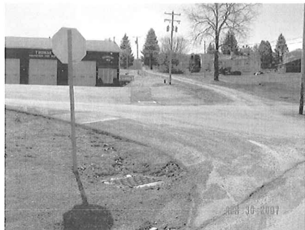
New Storm Drains and Catch Basins
