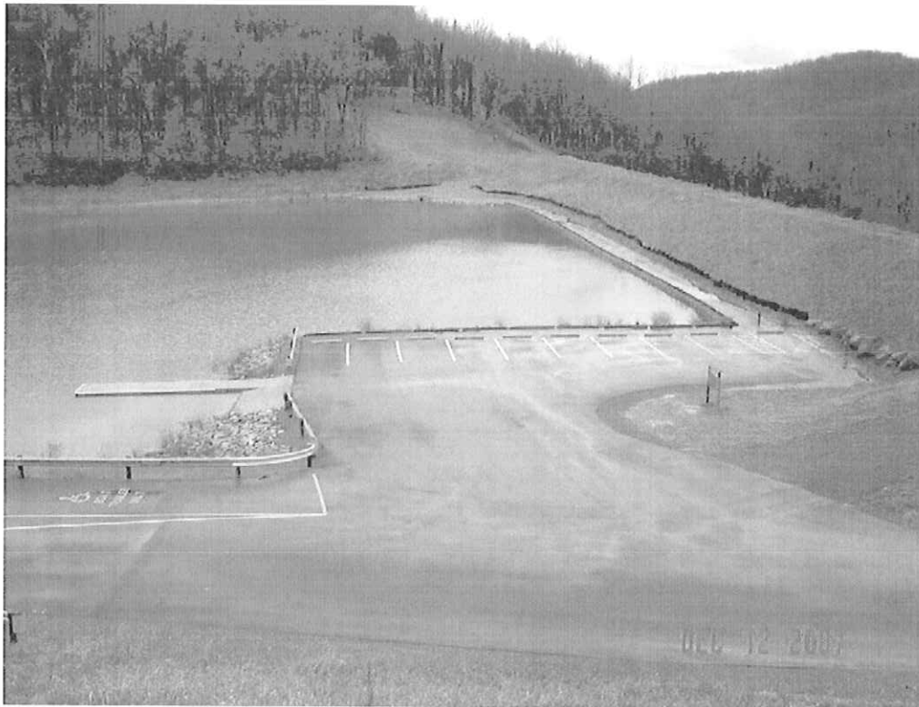
BAILEY DAM MODIFICATION, MONONGALIA CO., WV
