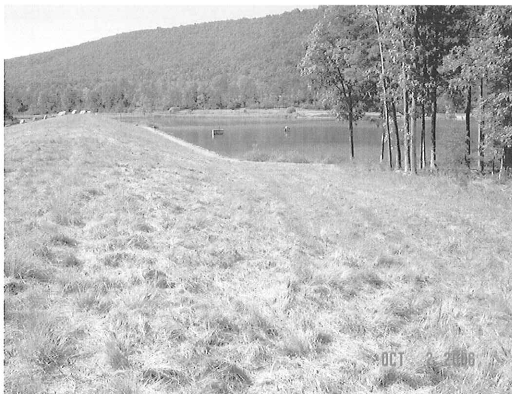
WARDEN LAKE DAM MODIFICATION, HARDY CO., WV
