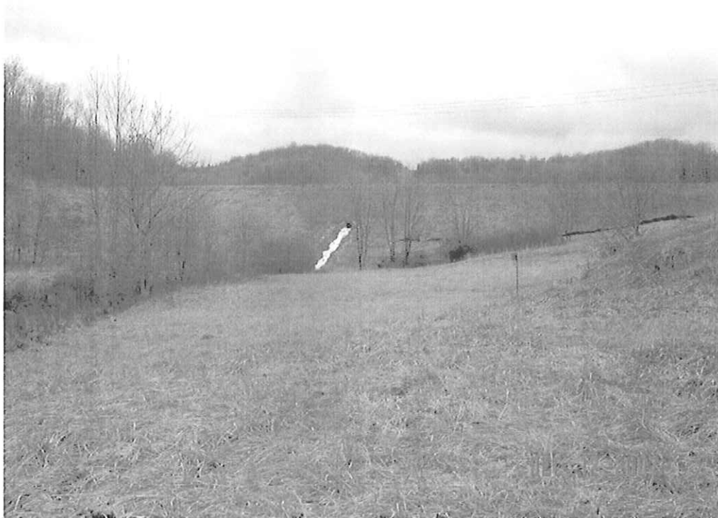
LEMLEY DAM MODIFICATION, MONONGALIA CO., WV
