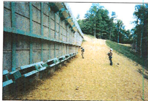
Finished wall with anchors
