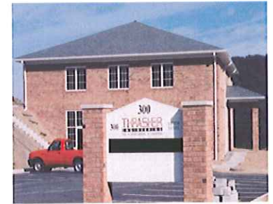
Thrasher Engineering, Inc. Office – Charleston, WV
