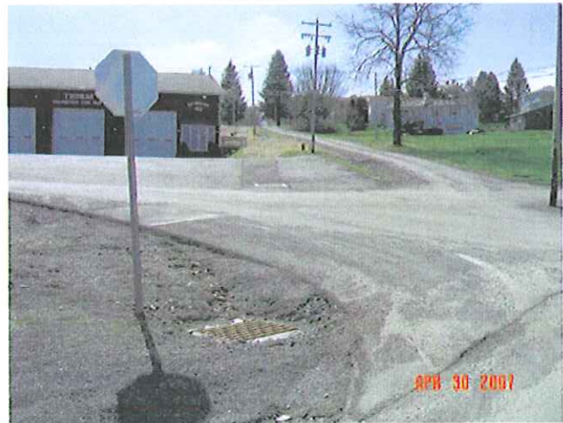
New Storm Drains and Catch Basins
