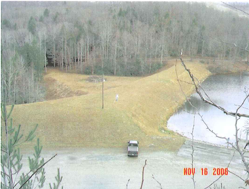
PLUM ORCHARD DAM MODIFICATION, FAYETTE CO., WV
