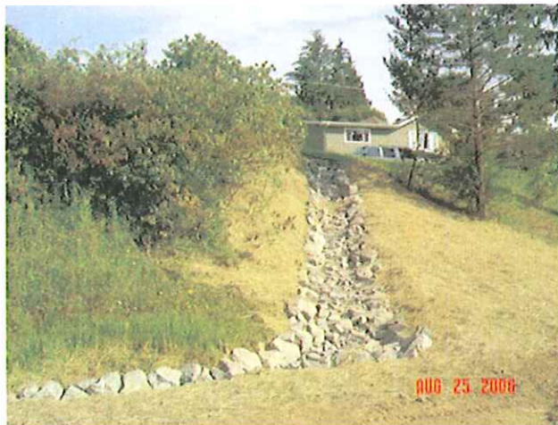
Erosion Repair – Rip Rap Armored Ditch
