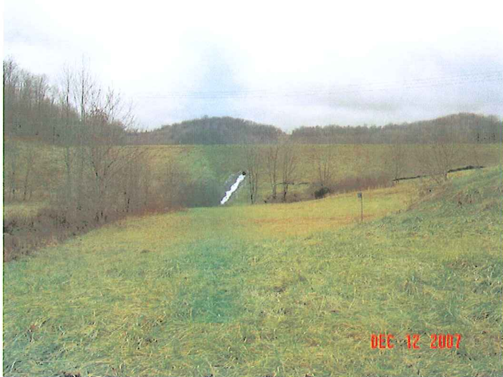
LEMLEY DAM MODIFICATION, MONONGALIA CO., WV
