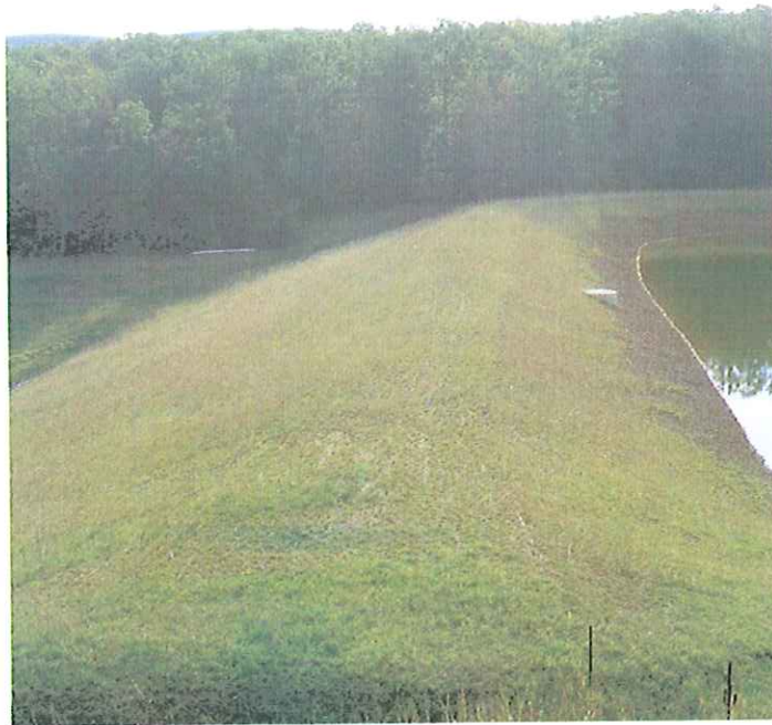
WILSON DAM MODIFICATION, HAMPSHIRE CO., WV
