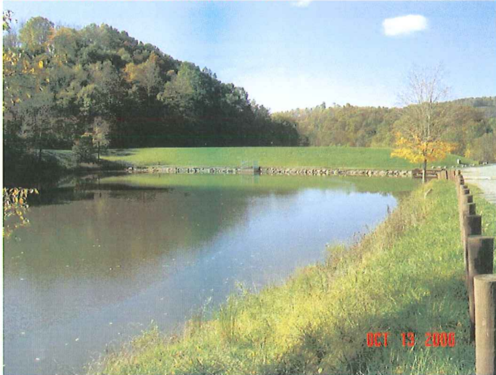
JIMMY LEWIS DAM MODIFICATION, MERCER CO., WV
