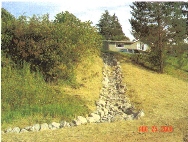
Erosion Repair – Rip Rap Armored Ditch
