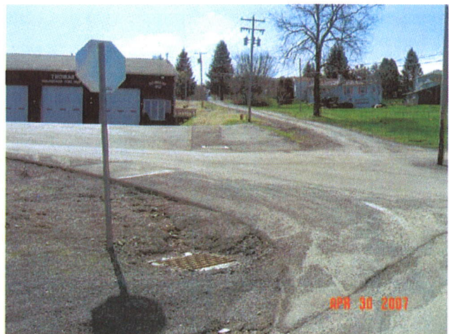
New Storm Drains and Catch Basins
