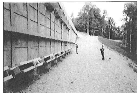
Finished wall with anchors
