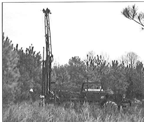
CTL's ATV can drill in rough terrain
