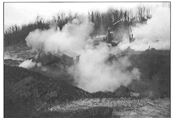
Jamison Burning Refuse Reclamation Project
