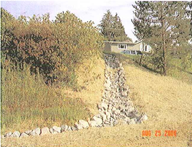
Erosion Repair – Rip Rap Armored Ditch
