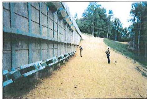
Finished wall with anchors
