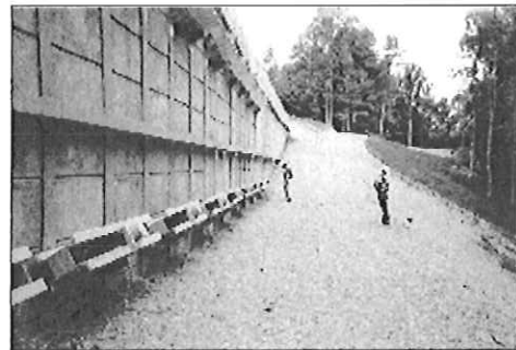
Finished wall with anchors
