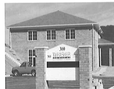
Thrasher Engineering, Inc. Office – Charleston, WV
