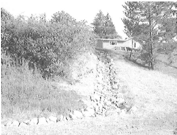
Erosion Repair – Rip Rap Armored Ditch
