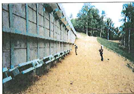
Finished wall with anchors
