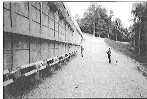
Finished wall with anchors
