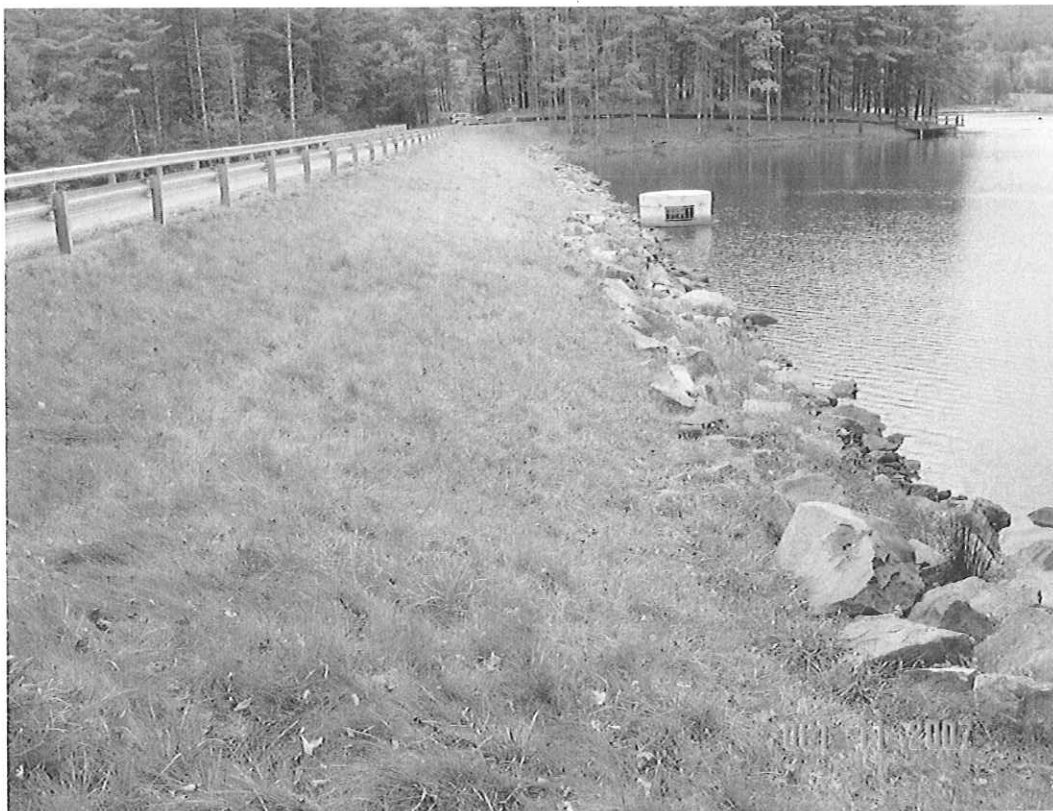
MONCOVE DAM MODIFICATION, MONROE CO., WV
