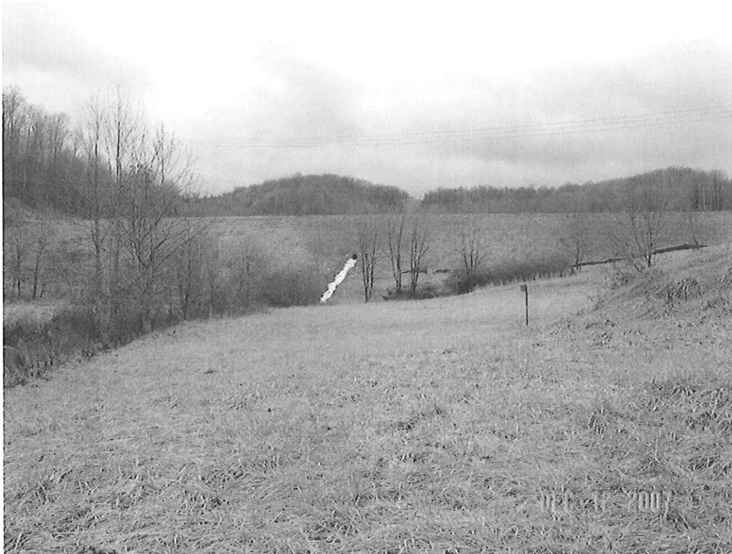
LEMLEY DAM MODIFICATION, MONONGALIA CO., WV
