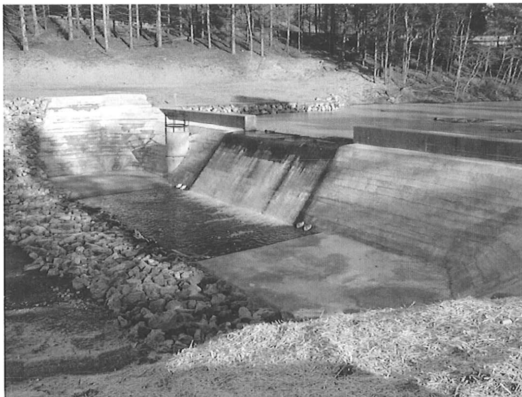
THOMAS DAM MODIFICATION, THOMAS, WV
