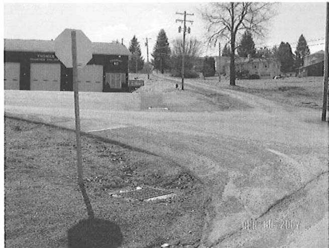
New Storm Drains and Catch Basins
