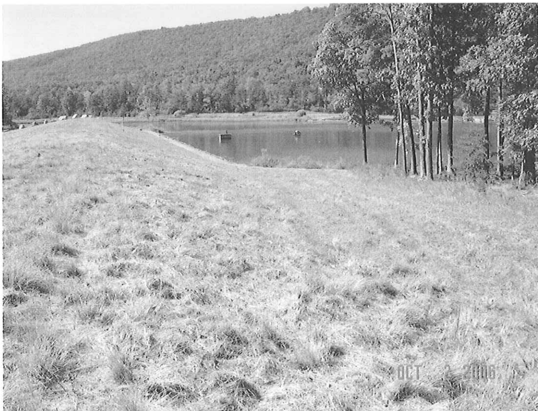
WARDEN LAKE DAM MODIFICATION, HARDY CO., WV
