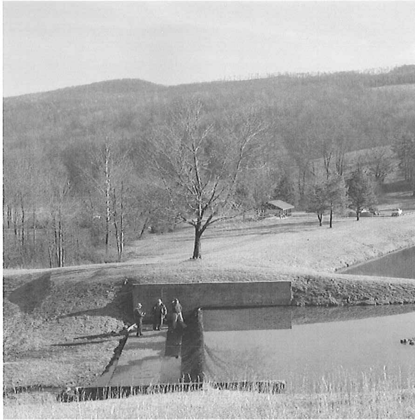
BELINGTON DAM MODIFICATION, BELINGTON, WV
