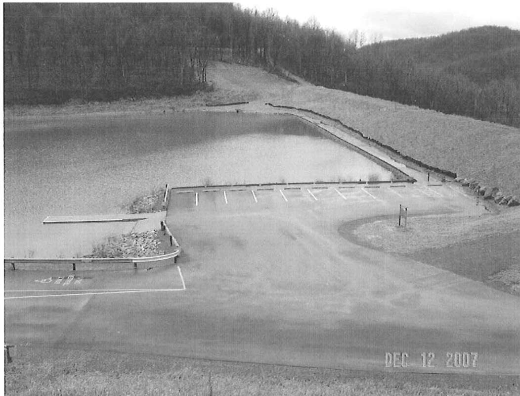
BAILEY DAM MODIFICATION, MONONGALIA CO., WV
