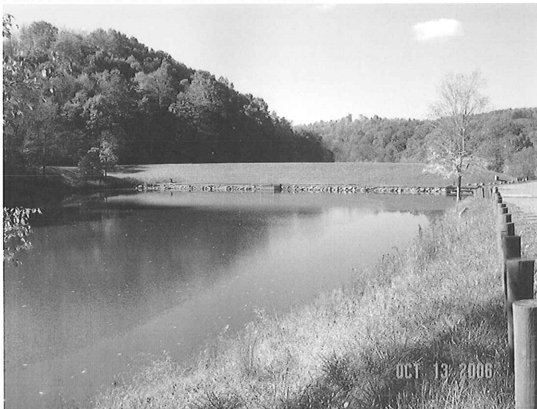
JIMMY LEWIS DAM MODIFICATION, MERCER CO., WV
