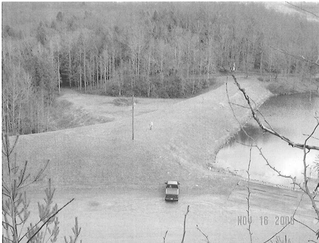
PLUM ORCHARD DAM MODIFICATION, FAYETTE CO., WV
