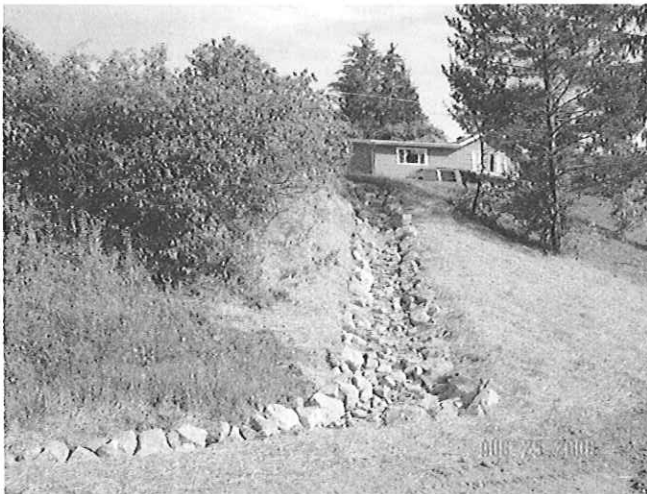
Erosion Repair – Rip Rap Armored Ditch
