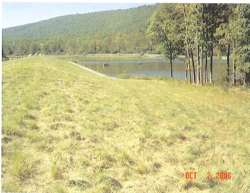
WARDEN LAKE DAM MODIFICATION, HARDY CO., WV
