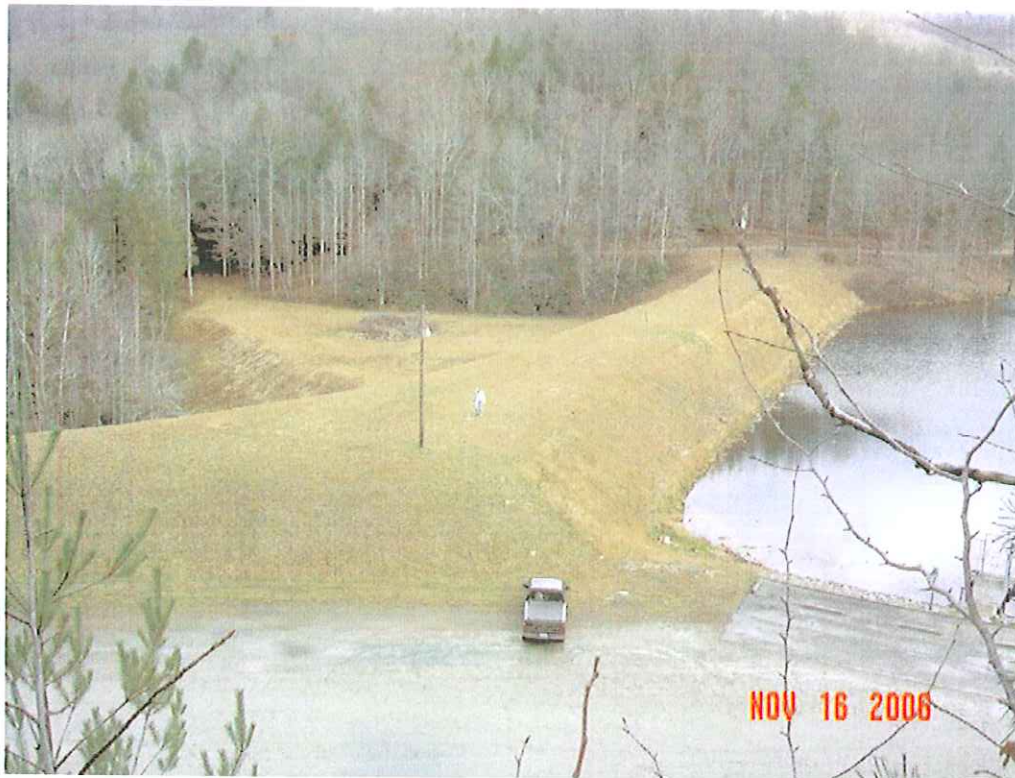
PLUM ORCHARD DAM MODIFICATION, FAYETTE CO., WV
