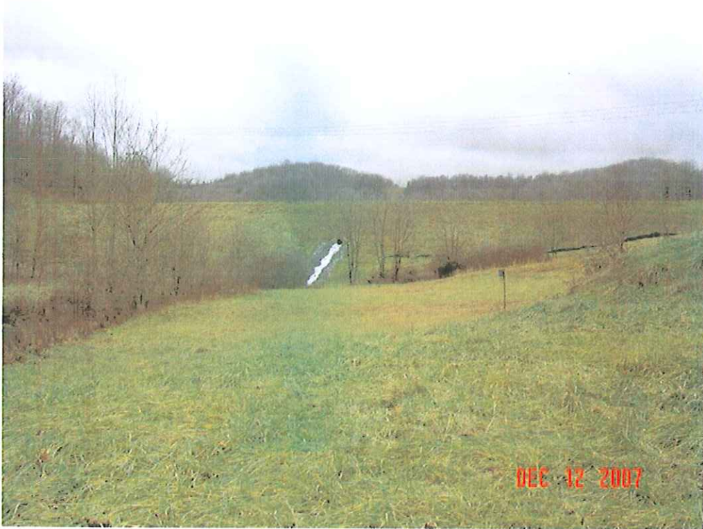
LEMLEY DAM MODIFICATION, MONONGALIA CO., WV
