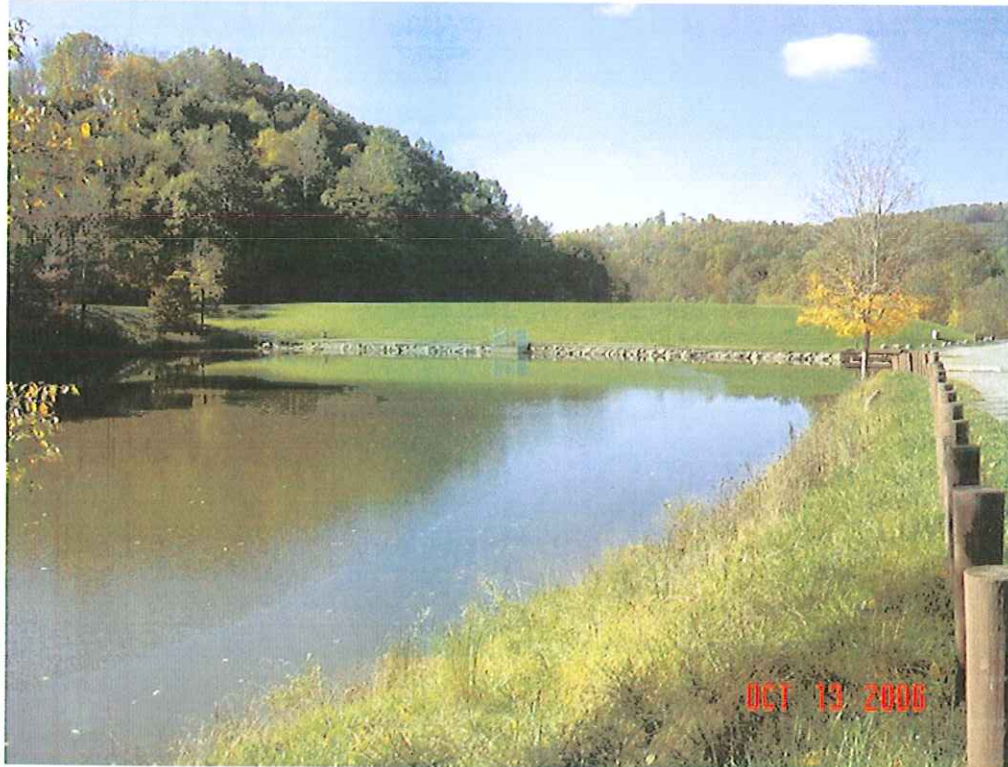
JIMMY LEWIS DAM MODIFICATION, MERCER CO., WV
