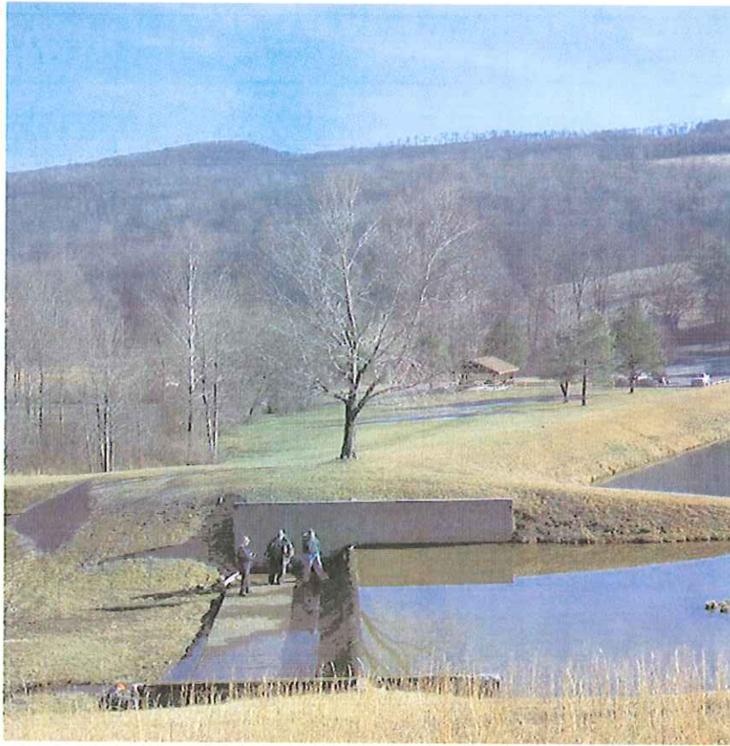
BELINGTON DAM MODIFICATION, BELINGTON, WV
