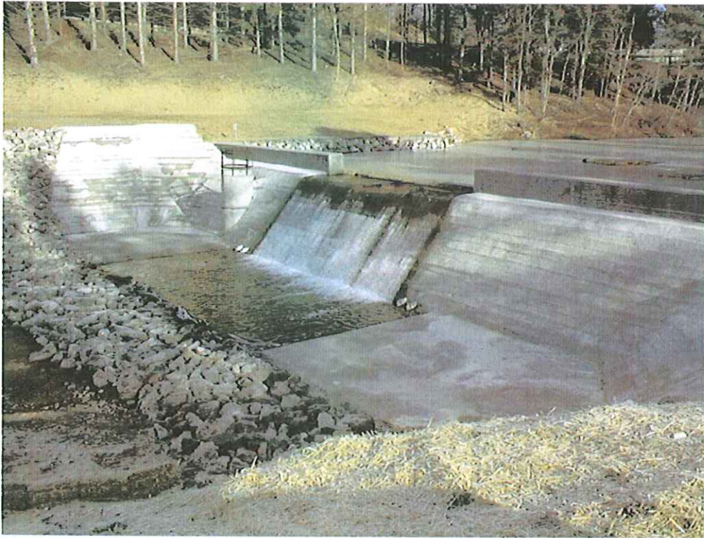
THOMAS DAM MODIFICATION, THOMAS, WV
