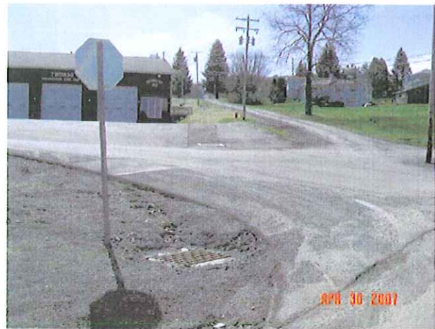
New Storm Drains and Catch Basins
