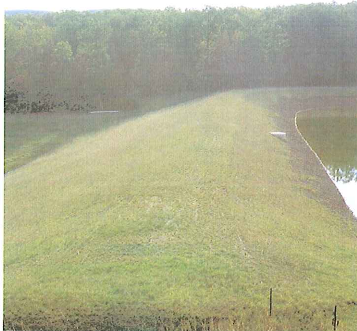
WILSON DAM MODIFICATION, HAMPSHIRE CO., WV
