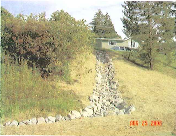
Erosion Repair – Rip Rap Armored Ditch
