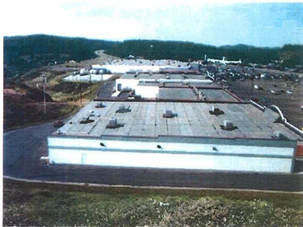
CTL Engineering of West Virginia, Inc. provided geotechnical engineering, materials testing, observation services and surveying services for this project.
