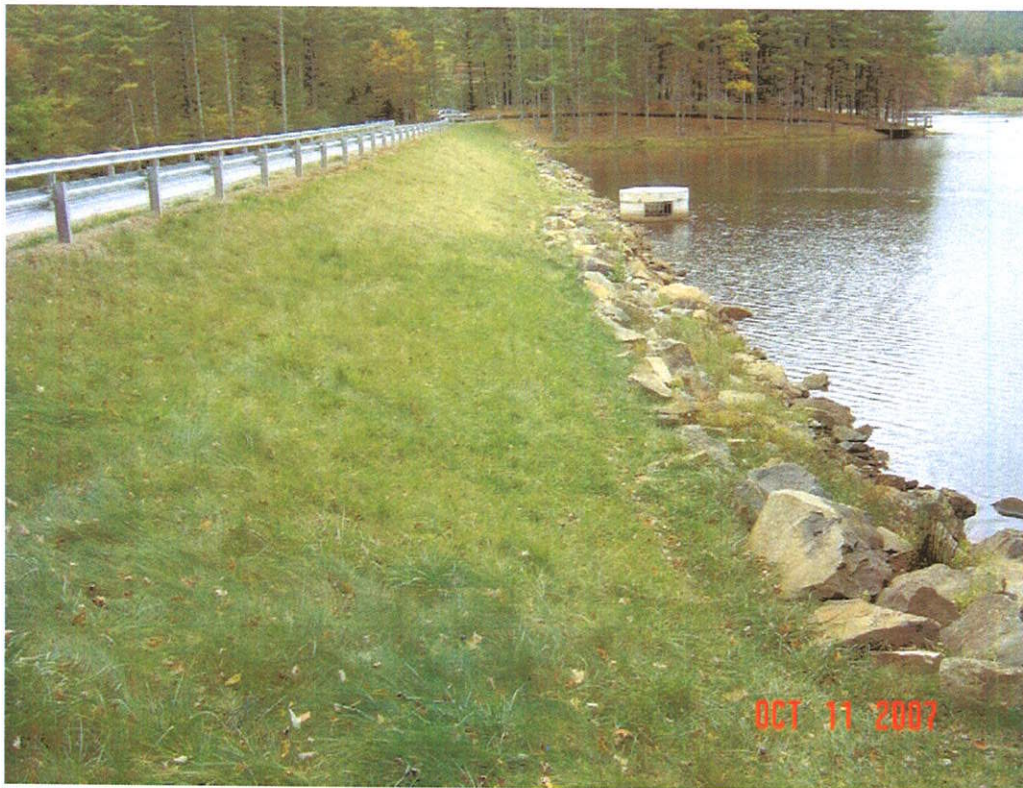
MONCOVE DAM MODIFICATION, MONROE CO., WV
