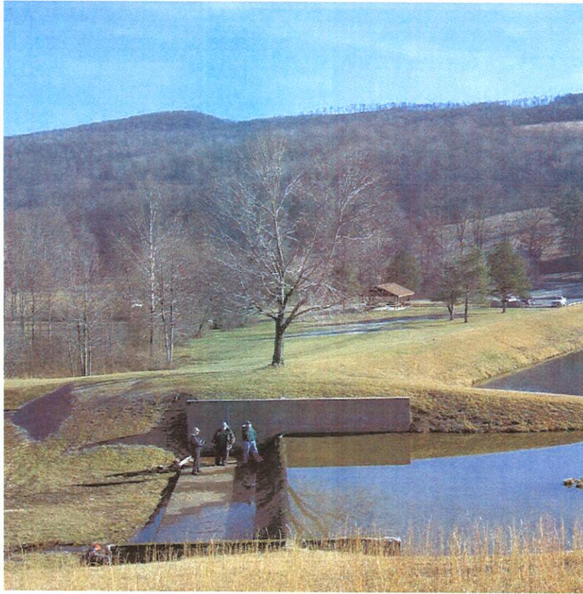
BELINGTON DAM MODIFICATION, BELINGTON, WV
