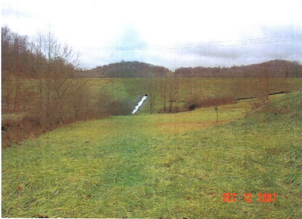
LEMLEY DAM MODIFICATION, MONONGALIA CO., WV
