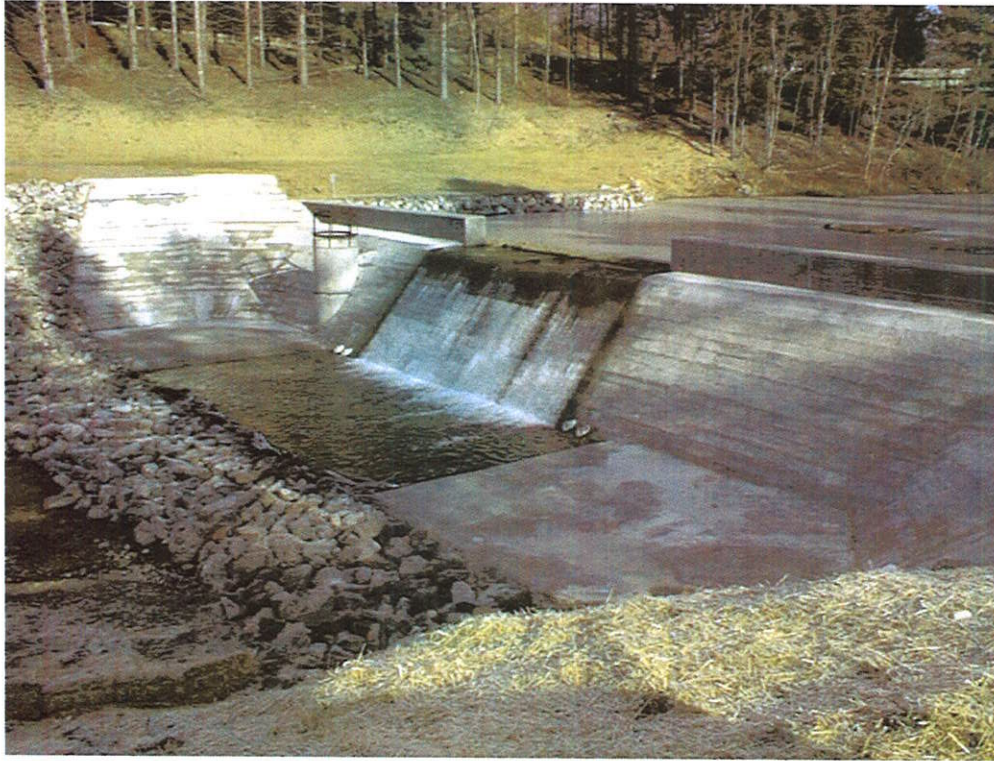
THOMAS DAM MODIFICATION, THOMAS, WV
