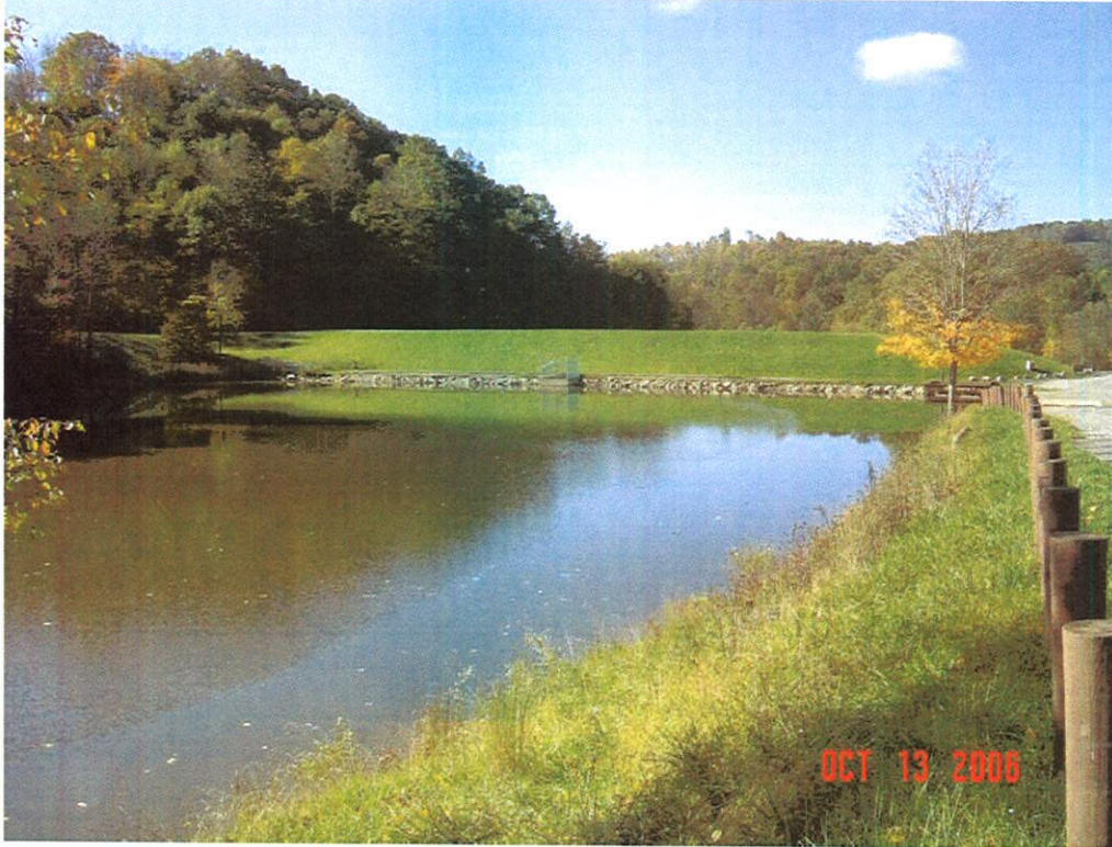
JIMMY LEWIS DAM MODIFICATION, MERCER CO., WV
