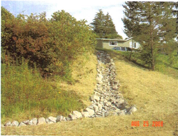
Erosion Repair – Rip Rap Armored Ditch
