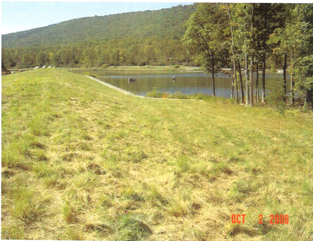
WARDEN LAKE DAM MODIFICATION, HARDY CO., WV
