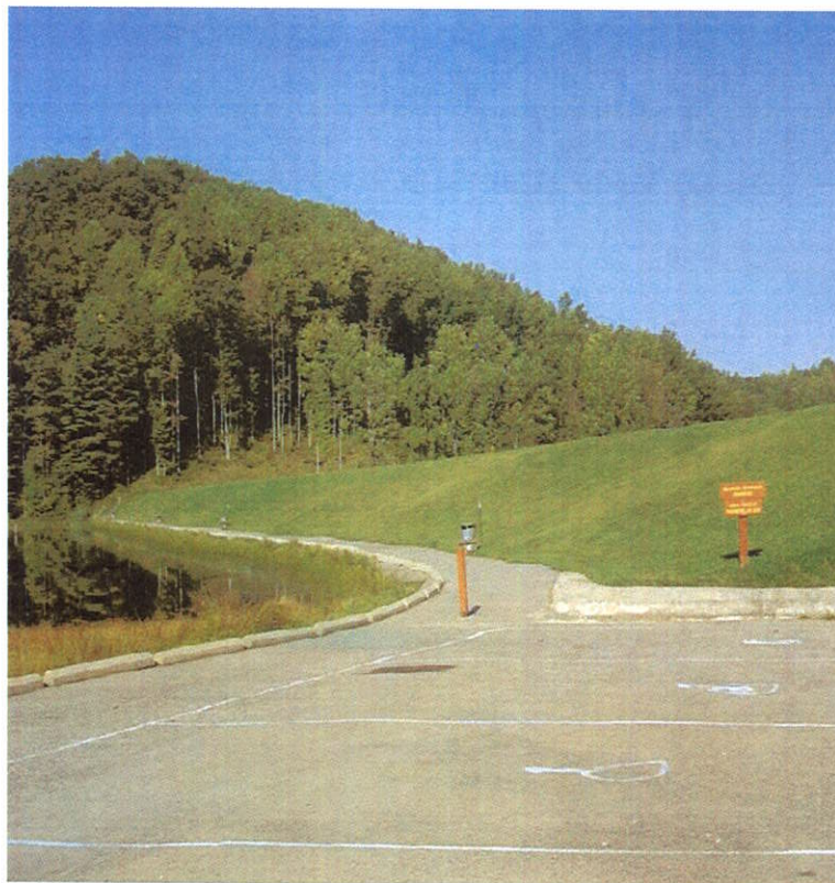
TETER CREEK DAM MODIFICATION, BARBOUR CO., WV
