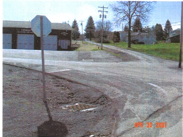
New Storm Drains and Catch Basins
