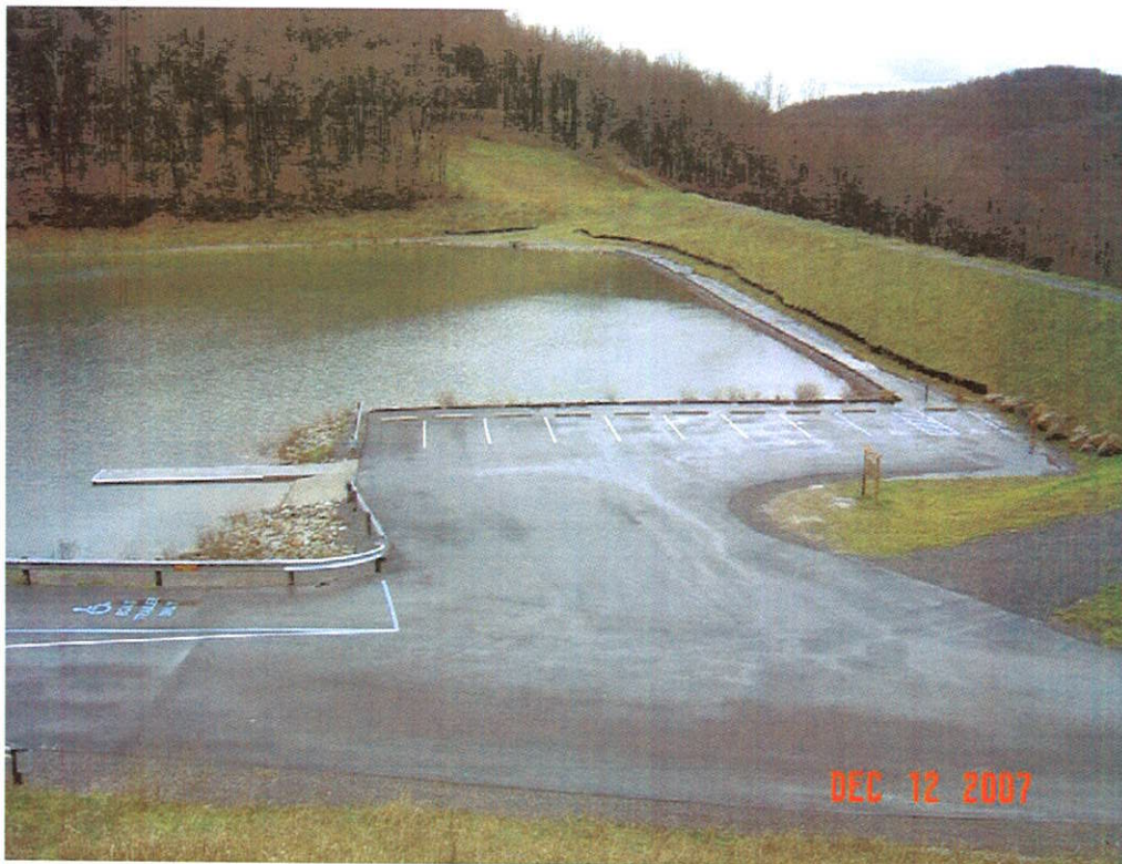
BAILEY DAM MODIFICATION, MONONGALIA CO., WV
