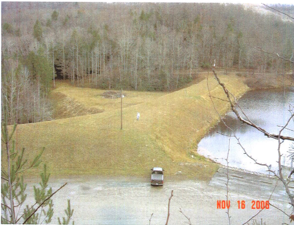
PLUM ORCHARD DAM MODIFICATION, FAYETTE CO., WV
