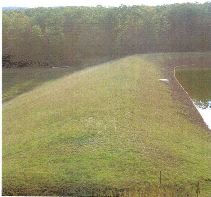
WILSON DAM MODIFICATION, HAMPSHIRE CO., WV
