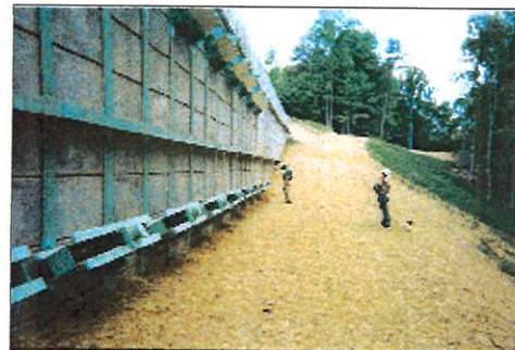
Finished wall with anchors
