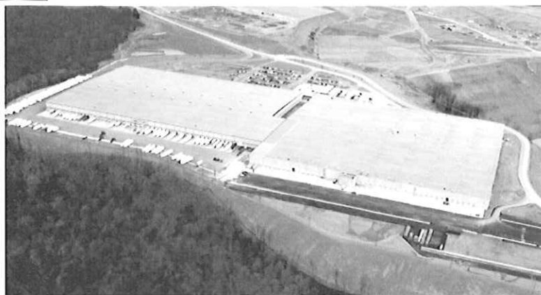
Cabela's Eastern Distribution Center
