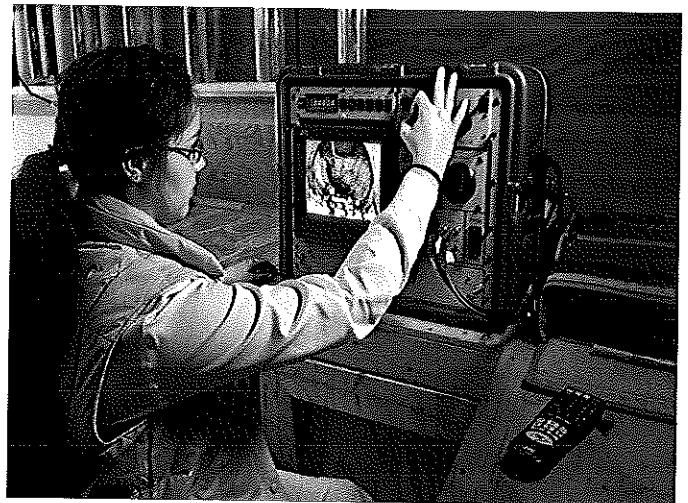
TEI's in-house Pipeline Inspection method includes video camera inspection. Results are available to clients on both VHS and DVD formats—Town of Reedsville
