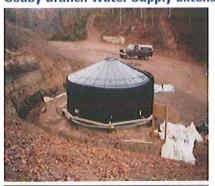
GAI was retained by WVDEP to design an extension and upgrade the Logan County Public Service District's public water system, involving a water line upgrade to offset decreases in pressure for existing low-press areas.
