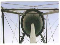
GAI was retained by Nextel Communications to perform structural analysis of the support legs and walkway platforms on an existing 130 foot high, 150,000 gallon capacity water tank for additional loadings associated with the installation of new communication antennas.
