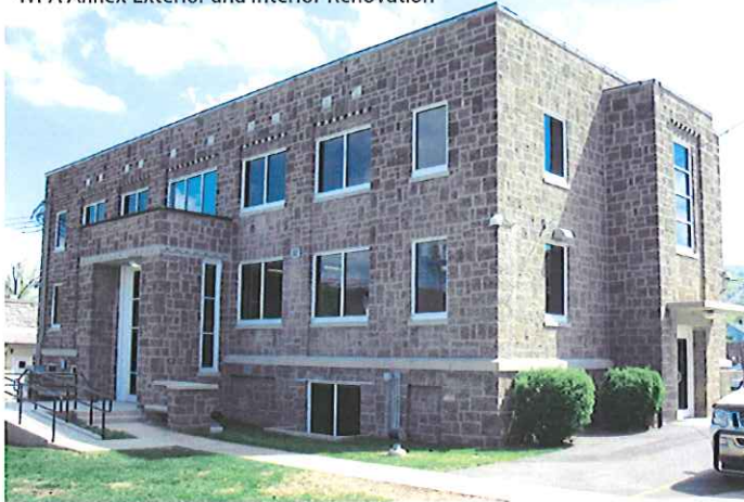
WPA Annex Exterior and Interior Renovation
