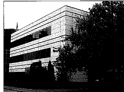
Pittsburgh & Charleston Offices
