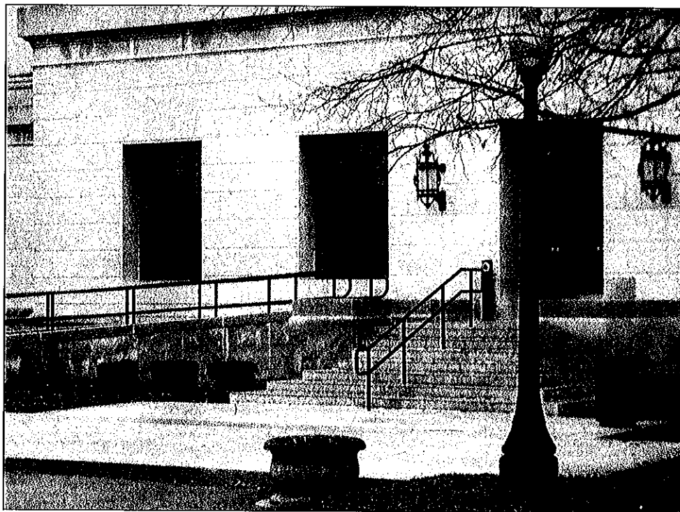
New West Entrance Stairs & Ramp
