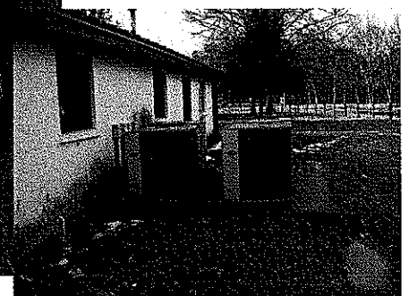
Outdoor HVAC Units
