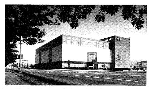
An existing three story Sears Roebuck retail facility was purchased by this client and completely renovated and expanded to provide space for corporate headquarters. A fourth floor of 25,000 SF was added, a significant structural engineering feature. The exterior of the building was clad in limestone and granite veneer with reflective glass windows and spandrel panels, masking the new floors presence.
